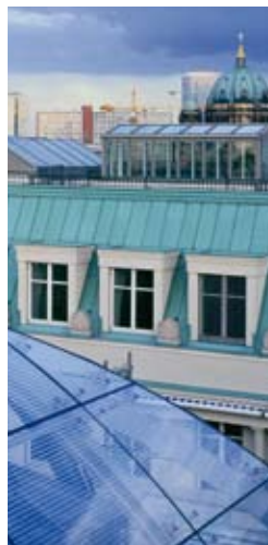
Sealing the glass façades
