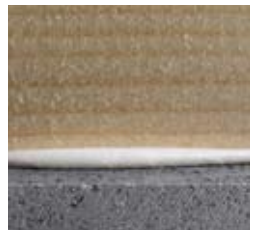
Wood on concrete
