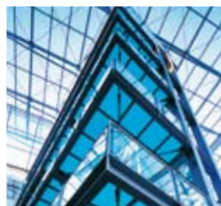
Sealing slanted glazing
