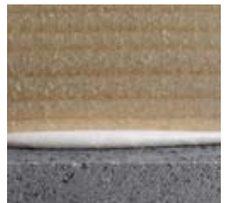
Wood on concrete
