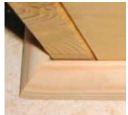
Wood strips on tiles
